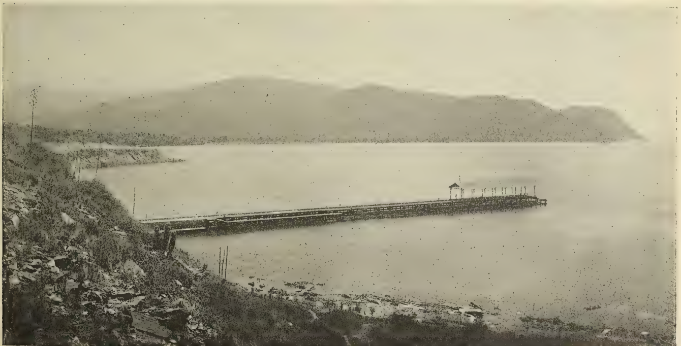
Newly Constructed Dock at Recently Opened Port of Ocumare de la Costa, Terminus of Spur from 1,800-Mile System of Modern Motor Highways
